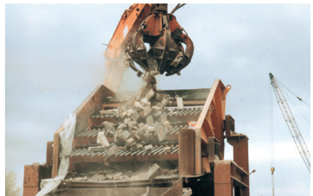
Model VS 2056 screening stone in construction project
